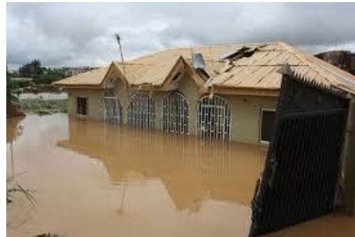
Plate 3. Home made inhabitable by flood water in Ibadan
