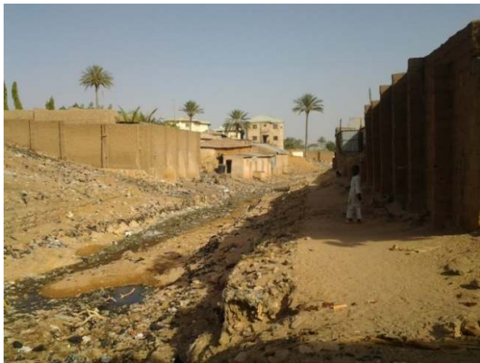
Fig. 1. Erosion path in residential area
